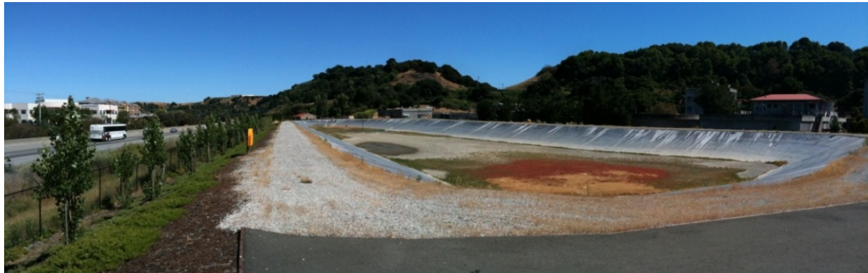
Effluent Storage Pond
