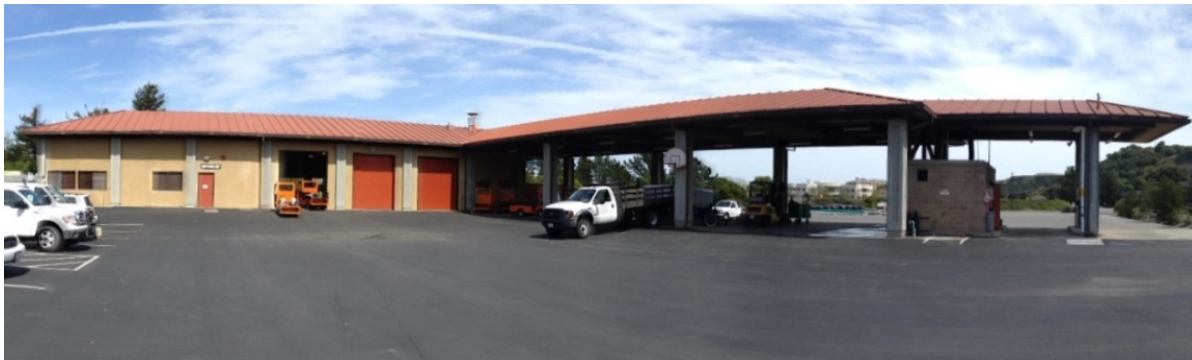
Maintenance Building with standing seam metal roofs
