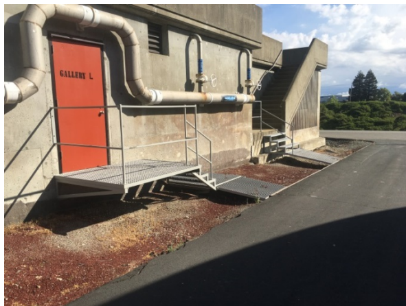
Stair modifications to account for settlement
