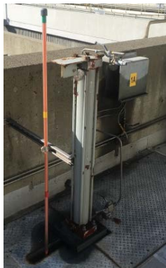
Hydraulic gate actuator
