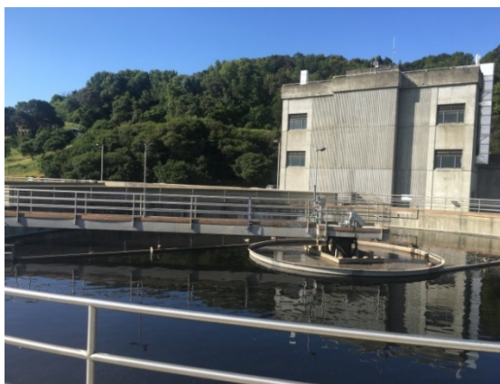
Secondary clarifier in operation
